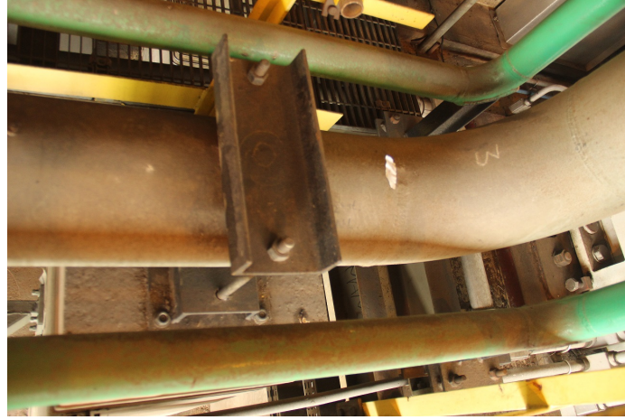
Figure 5.42: Intermediary pipe support.
